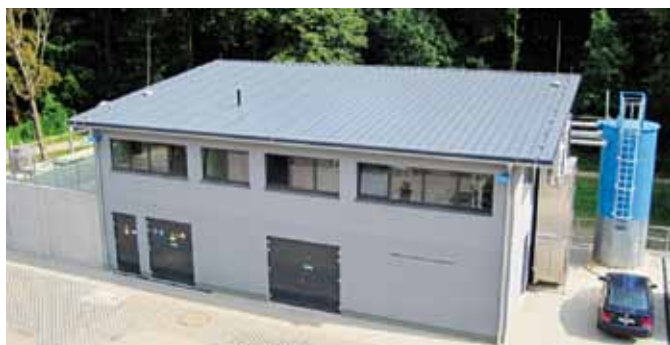
The hospital waste water treatment facility of the Emschergenossenschaft at Marienhospital Gelsenkirchen (D)
